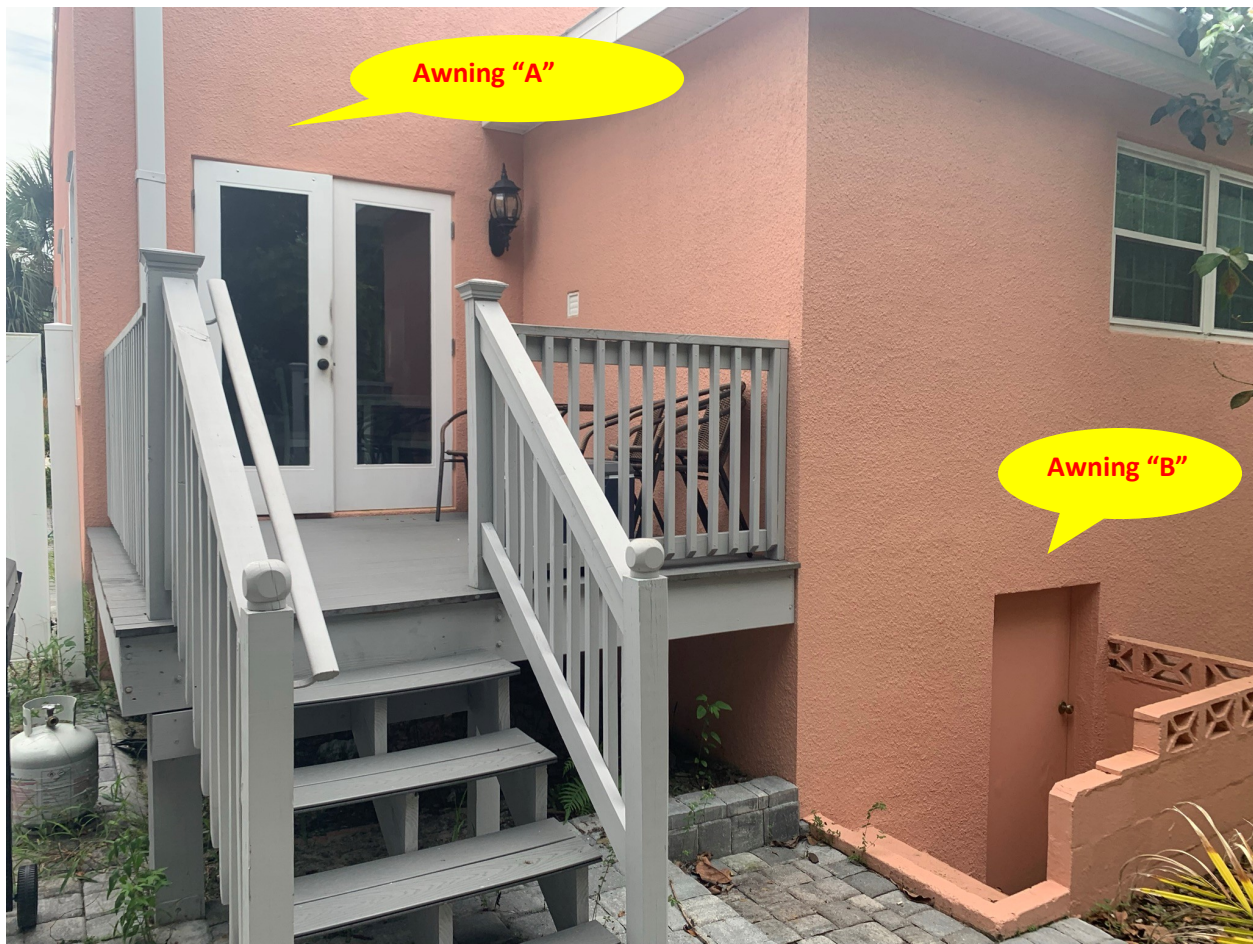
Figure 7 Rear of 211 Jessamine with awning locations
