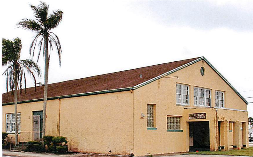
Figure 2 - 110 E Orange Avenue "Rec Center"
